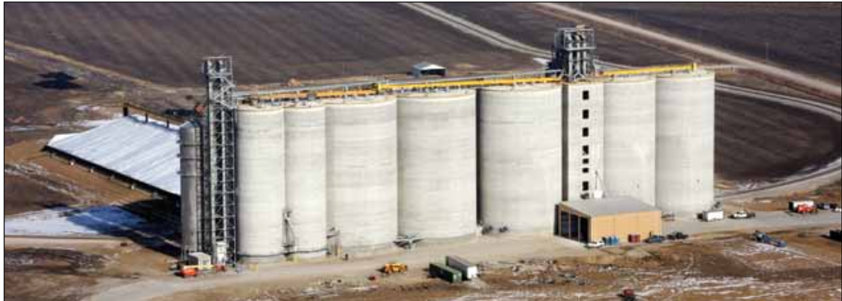
DeBruce Grain Inc.'s new 6.4-million-bushel rail terminal in the Missouri River bottom land near Rock Port, MO began taking in grain and loading railcars in September 2010. Aerial photo by JH Photography, Spencer, IA.
