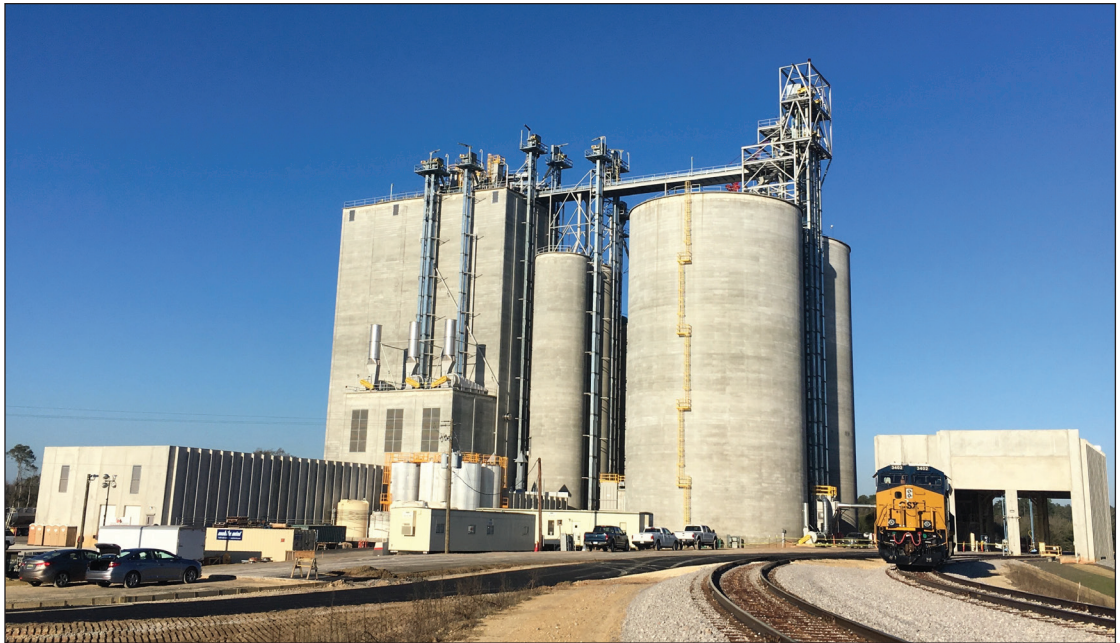
Wayne Farms' new 25,000-tpw poultry feed mill in Ozark, AL features three receiving systems, two 500,000-bushel concrete storage silos, two batching systems, and three pelleting lines. Photo courtesy of Wayne Farms LLC.
