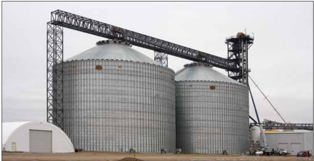
New steel annex at Fullerton Farmers Elevator in Fullerton, ND includes two GSI 1.2-million-bushel steel tanks and a pair of 20,000-bph receiving legs. Photos by Judy Hemphill, JH Photography, Spencer, IA.
