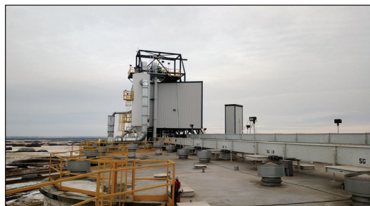
Rooftop view looking toward the facility cleaning house, leg head sections, and a manlift, as well as VIS 23,000-bph drag conveyors.
