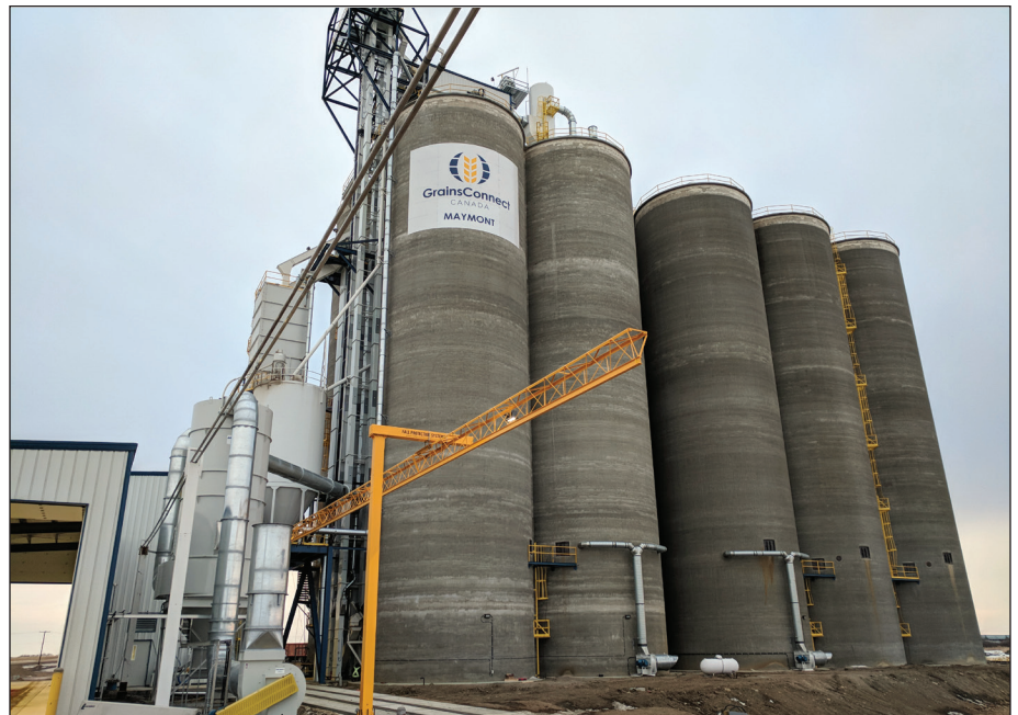
Ground-level view of the terminal shows a slipform concrete 10-pack of storage tanks. Not visible are 12 additional interstice bins. Ground photos courtesy of Todd & Sargent Inc.
