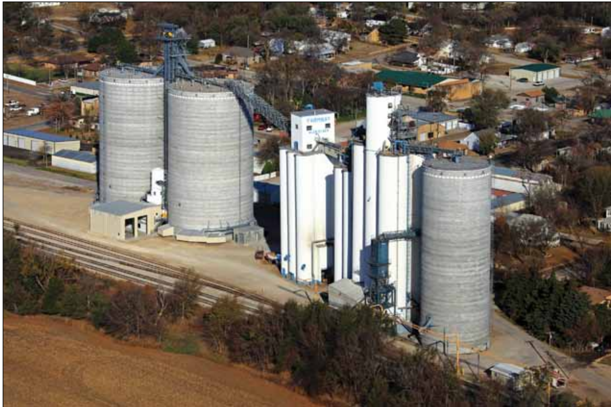
Expansion project at Farmway Coop in Glen Elder, KS includes two McPherson jumpform concrete tanks at left, Intersystems receiving legs and Hayes & Stolz distributor visible between tanks, and a pair of covered receiving pits in front of tanks. Aerial photo courtesy of McPherson Concrete Storage Systems, Inc.
