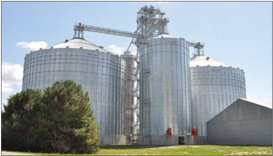
Farmers Pride Cooperative's flagship elevator at Neligh, NE, with three new corrugated steel storage tanks in foreground and a new tower dryer visible between the tanks. Photos by Ed Zdrojewski.
