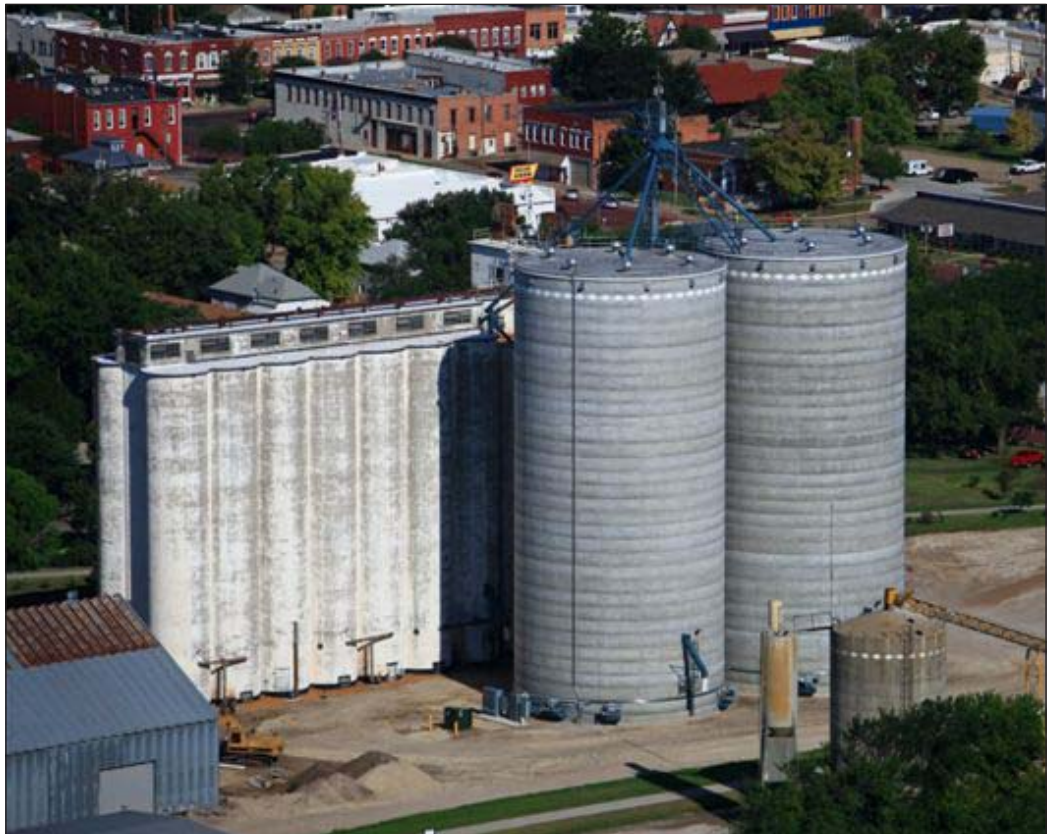
Mid Kansas Coop Association's grain elevator at Lindsborg, KS, with two new McPherson jumpform concrete tanks holding 318,000 bushels each at right. Aerial photo courtesy of McPherson Concrete Storage Systems.
