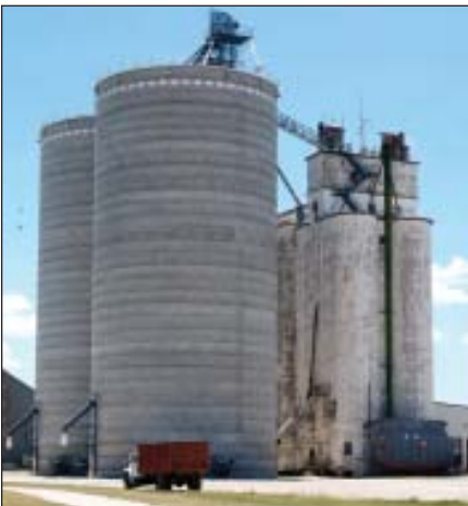
Ground level view of the new McPherson concrete storage tanks.
