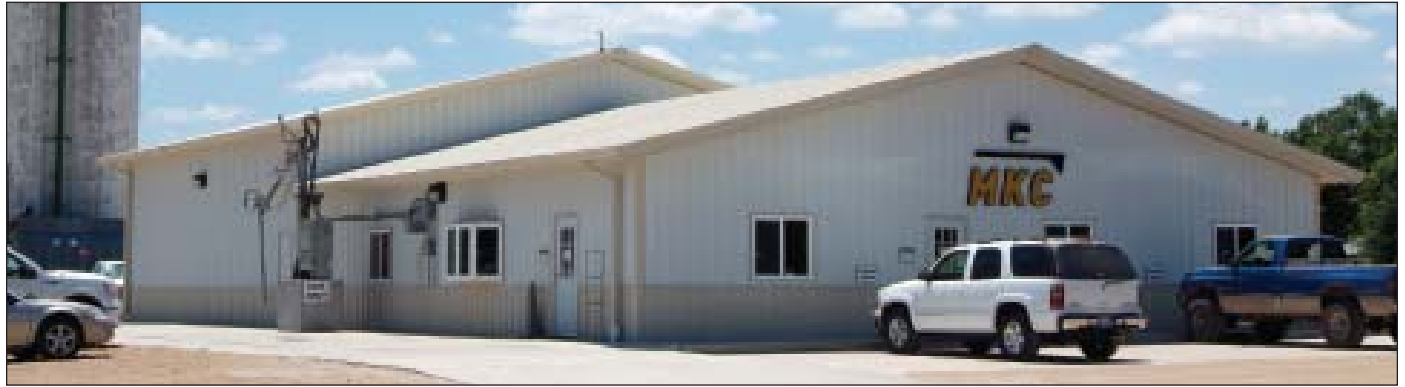
New regional office building for Mid Kansas Coop Association at Lindsborg, including new 80-foot-long truck scale from Salina Scales and Intersystems truck probe at left. Ground-level photos by Ed Zdrojewski.
