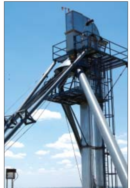
New 19,400-bph Intersystems leg feeds into a six-hole Schlagel rotary distributor.
