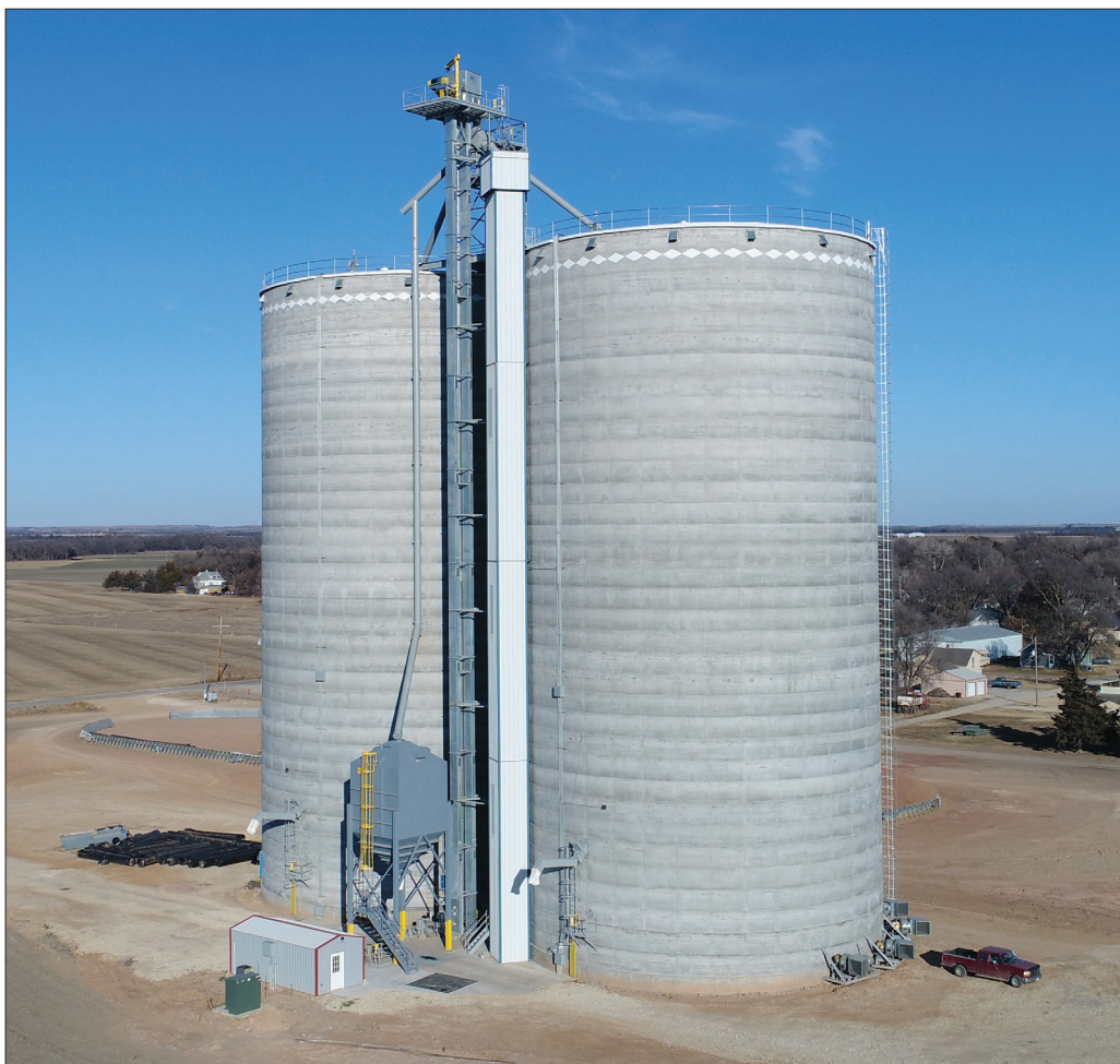
Delphos Cooperative Association's new 1-million-bushel annex about a quarter mile away from its headquarters facility in Delphos, KS. Drone photo courtesy of McPherson Concrete Storage Systems.
