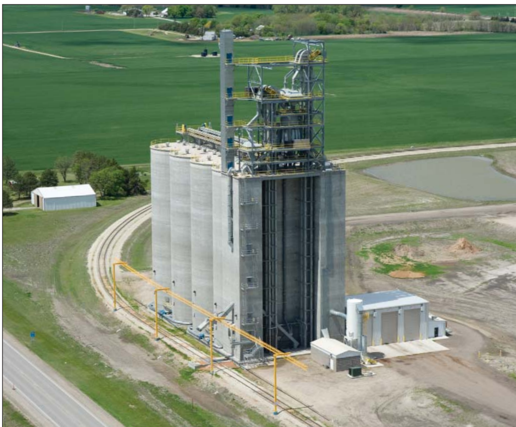
Producers Ag LLC's new 1.1-million-bushel slipform concrete elevator outside of Canton, KS nearing completion in November 2014. Aerial Photo by Steve Brown Photography, Wichita, KS.
