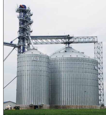
Center Valley added a GSI 105,000-bushel wet bin (left) and a GSI 618,000-bushel dry storage bin, two Schlager legs in a 174-foot tall Warrior support tower.
