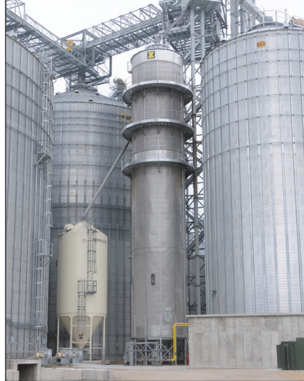
One of two new Zimmerman 4,750-bph tower dryers at Readfield. A third, identical dryer was added at Center Valley.
