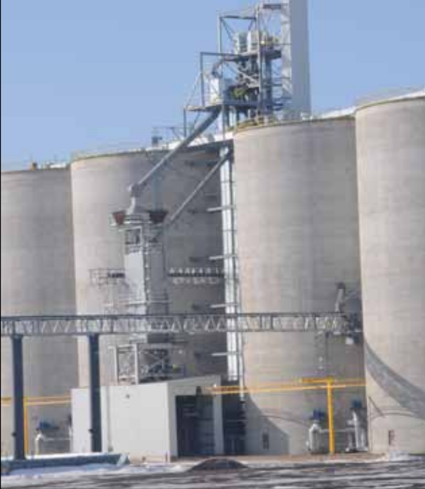
The facility can load railcars and trucks simultaneously at up to 80,000 bph.
