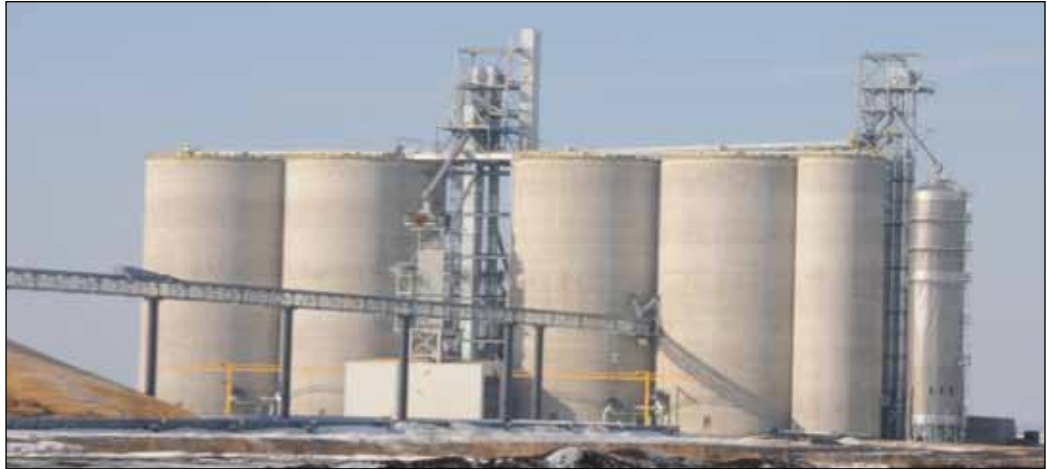
Gavilon's new Warren, IL train-loading terminal has a 4.2-million-bushel-capacity, with a target speed of unloading trucks and loading railcars at four minutes each. Photos by Stu Ellis.
