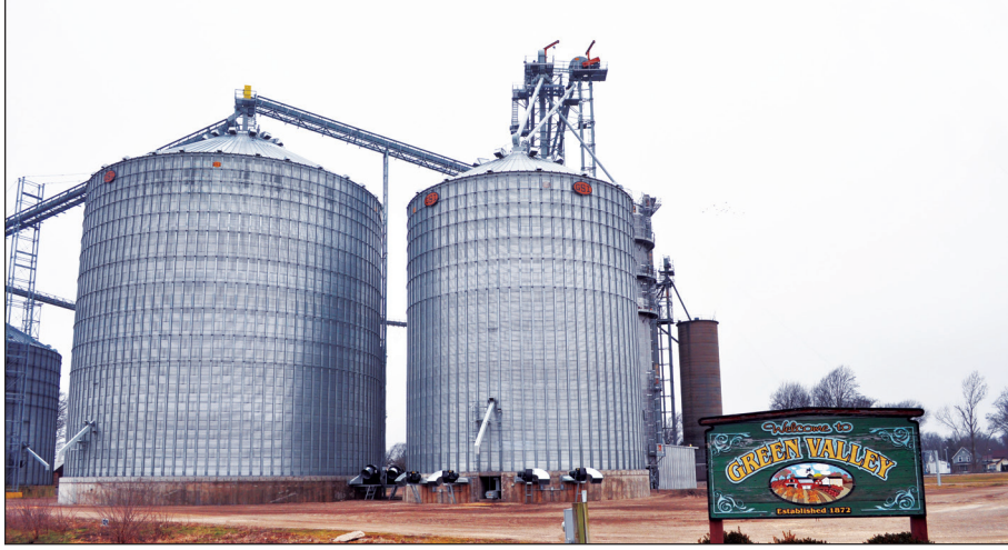
Western view of the 1.2 million bushels of new steel storage at the west end of Green Valley.
