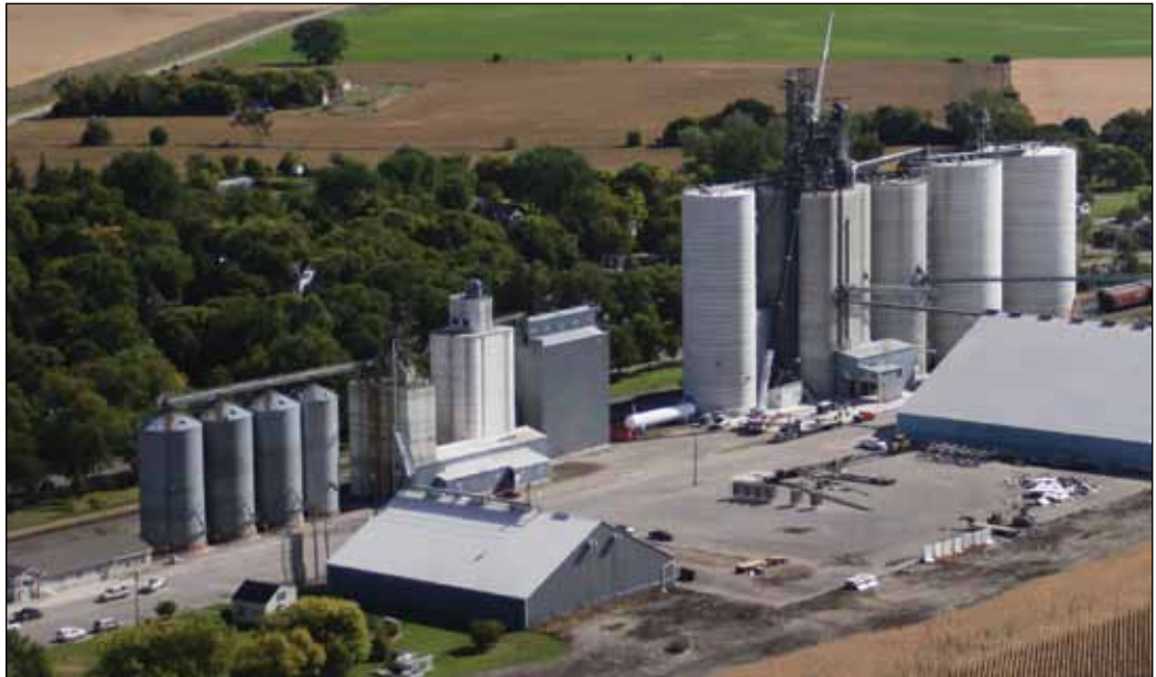
A new 450,000-bushel jumpform concrete silo built at Glacial Plains Cooperative at Murdock, MN in 2011 is visible at the far right. Aerial photo taken by R. DuMont/New Horizons Aerial Photography.
