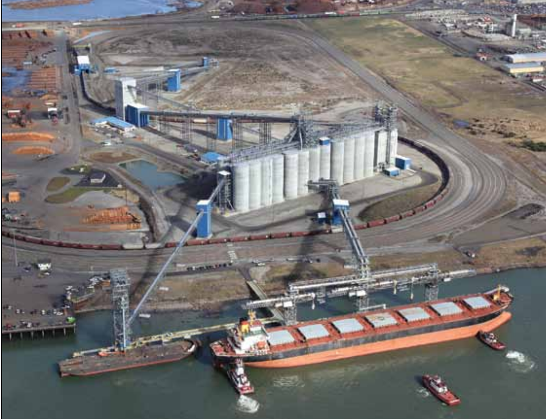
Aerial view of the EGT export complex at the Port of Longview includes roughly 11 miles of track, which has enough space to park four fully-loaded 110-car shuttle trains plus two empty trains awaiting departure. Aerial photo courtesy of EGT, LLC.
